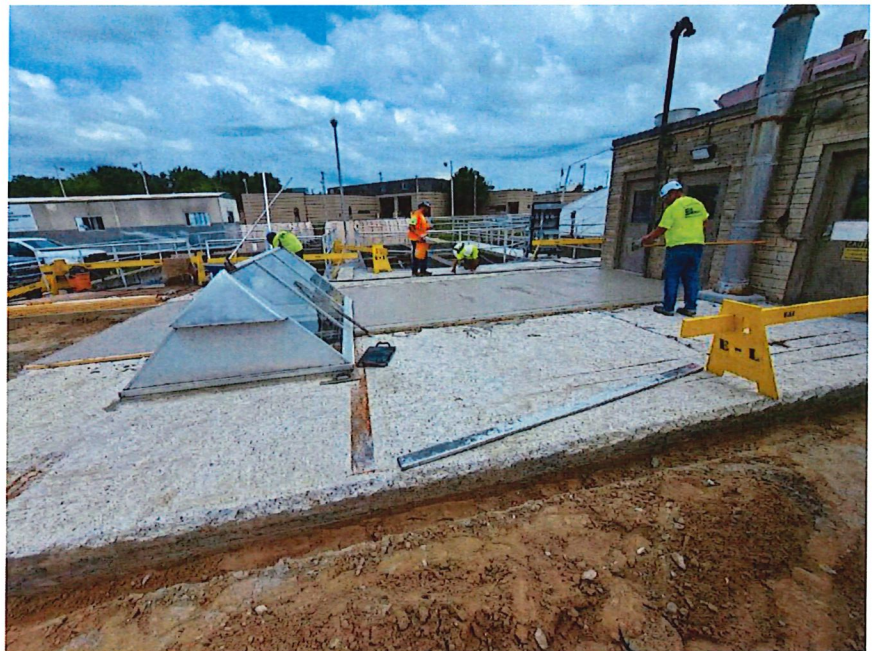
Figure 5 Primary Tank Deck Concrete Repair
